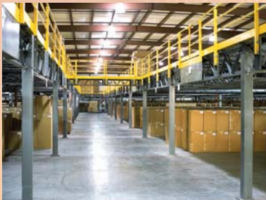
Warehouse Mezzanine with Walkway Bridge
