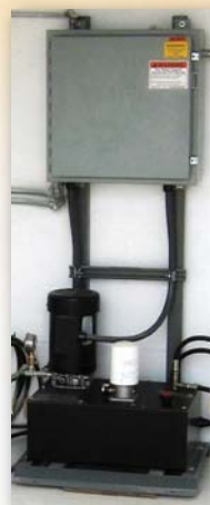
Hydraulic Pump System with control panel
