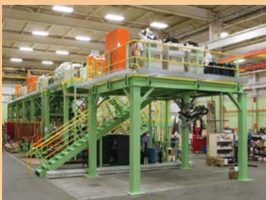
Manufacturing Mezzanine with Gantry Robot
